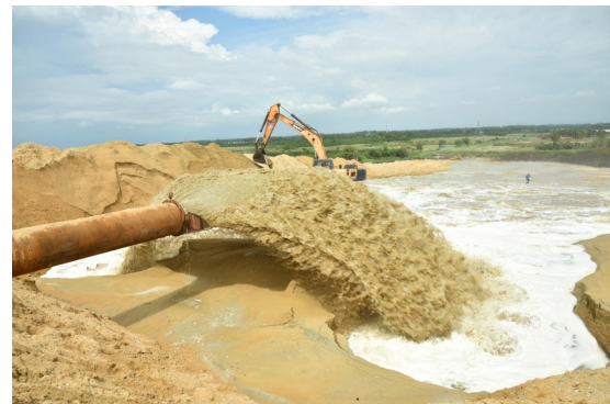
Figure 1 - Offshore sand pumping
