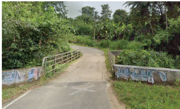
Fig. 2. A view of the Madulla bridge before failure
